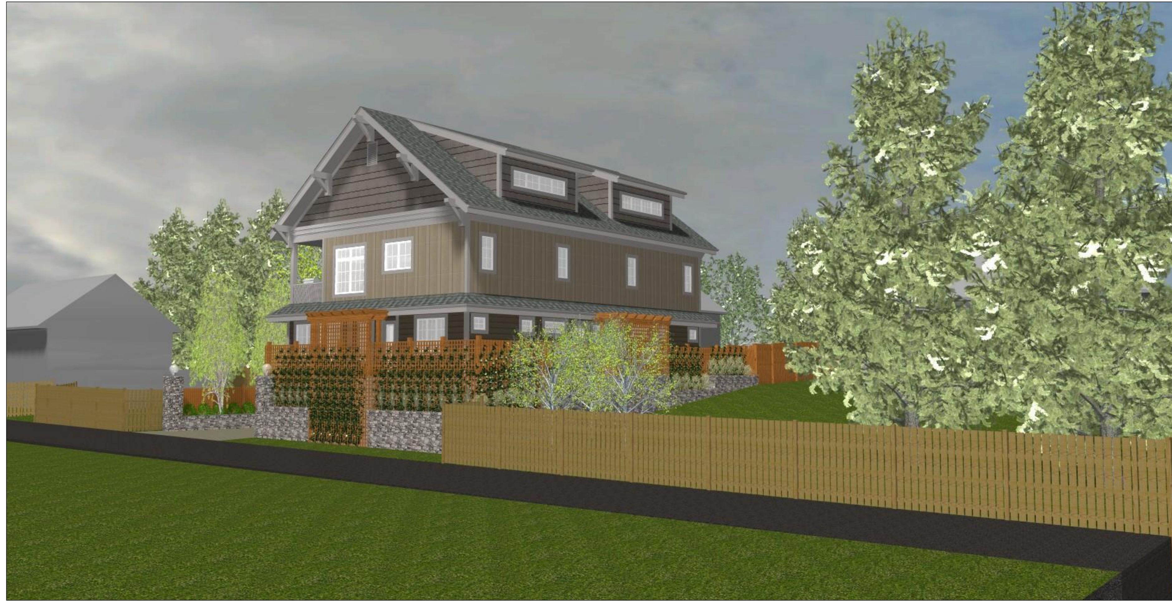
SOUTH LOOKING NORTH FROM MACHLEARY LANE
